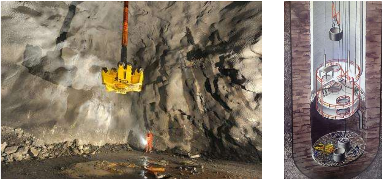
Figure 11.: Methodology of making shafts: "raise boring method" (left) and method of lowering shafts ("shaft sinking").
