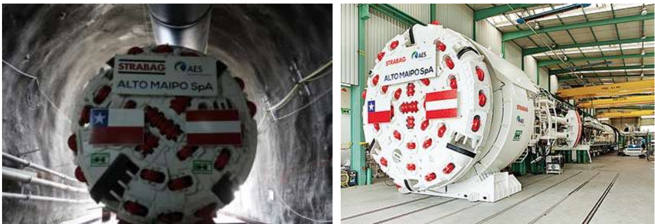
Figure 7. TBM for tunnel L1 tunnela Las Lajas and side view by start-up mounting in production facility.
