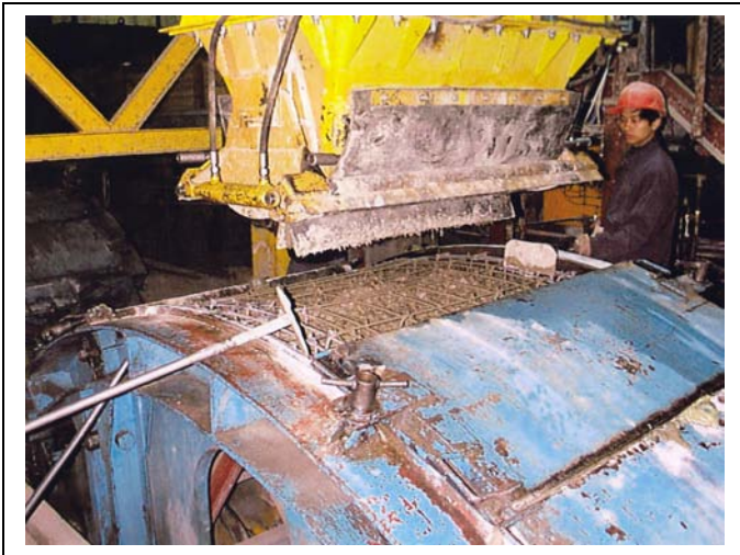
Figure 6. Concreting of segments in the hall of casting yard.
