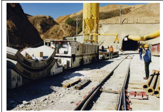
Figure 9. Supply train bringing segments toward tunnel face.
