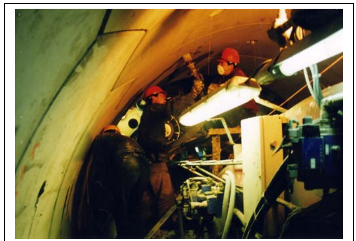
Figure 11. Filling the lining gap with the pea-gravel.
