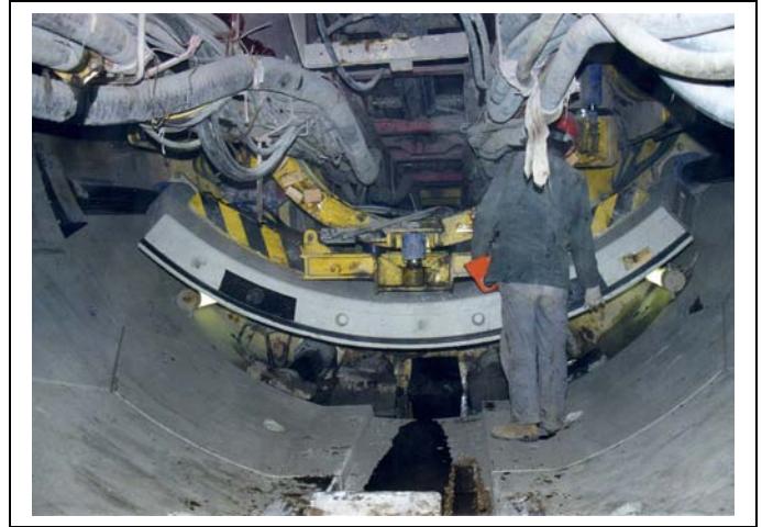
Figure 10. Segment installation within the shield tail.
