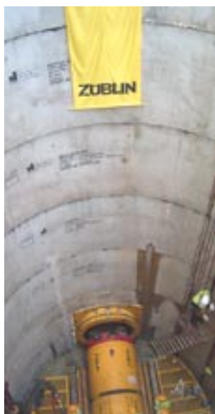
Figure 10: AVN 1200 pipe jacking equipment mounted in the start shaft.
