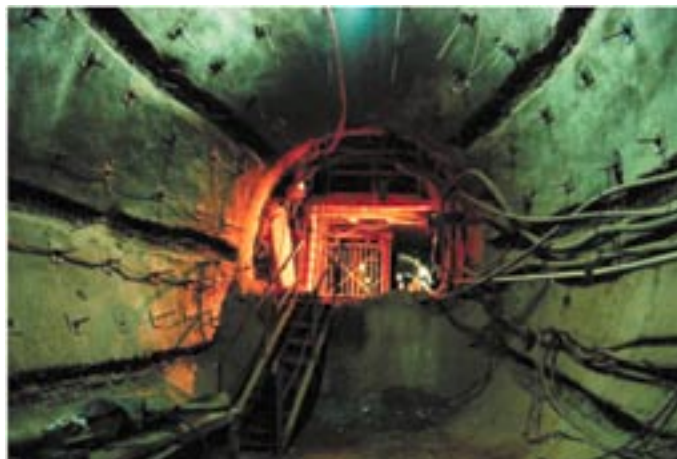
Figure 5. Shotcrete method in squeezing rock, deformable lining.
