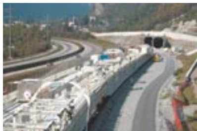
Fig. 14: Portal Bodio, lining installations before moving into the opencast constructed tunnel.
