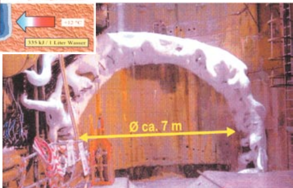
Nitrogen freezing viewed from the portal wall of the tunnel.
