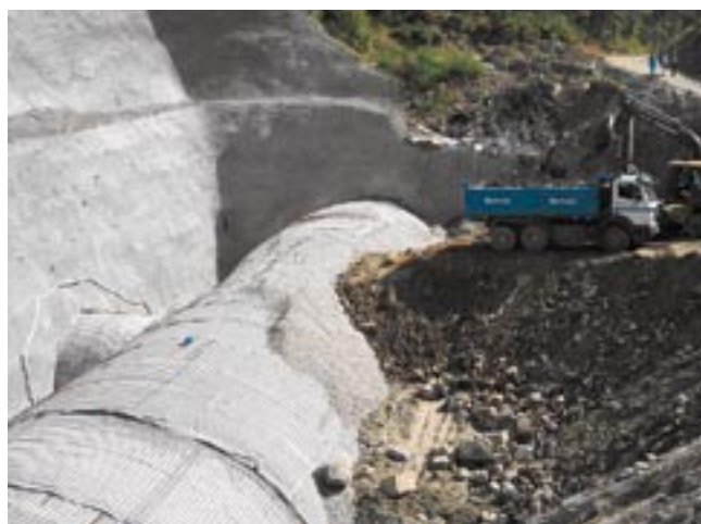
Figure 7: Deposition of material at Zamatavinec »cut and cover« reinforced structure
