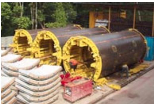
Figure 6: Shutters for the Secondary Lining.
