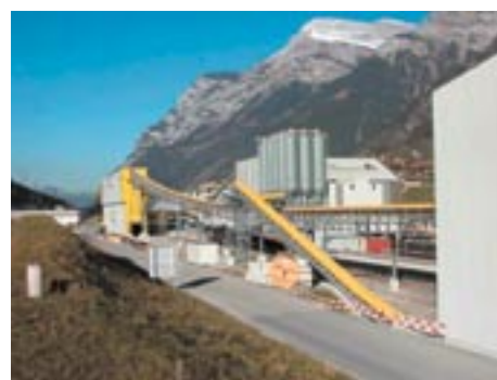
Fig. 20: Construction site Amsteg, encapsulated plants and conveyors belt systems.
