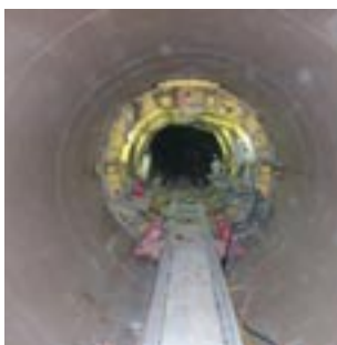
Figure 7: CPL Lining inside the Tunnel
