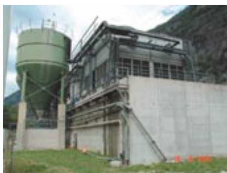
Fig. 19: Construction site Bodio, treatment of wastewater from the tunnel.
