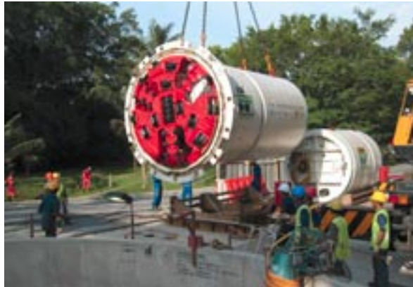
Figure 11: Dual Mode Pipe Jacking machine for ID 2400 Section.
