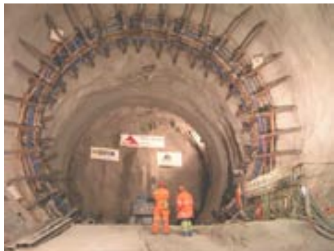
Fig. 9: Tunnel Sedrun, tests for yielding lining.
