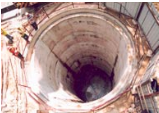
Figure 9: Shaft Sinking at the UTLS Project.
