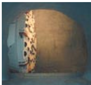
Fig. 7: Tunnel Amsteg, east tube, TBM cutter-head TBM.
