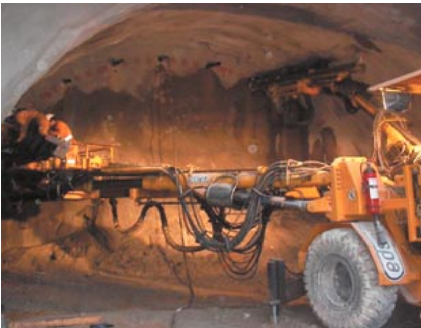
Fig. No. 2 Drilling of the micropiles umbrella
