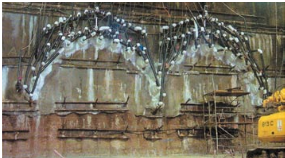
Tunnel with brine freezing methode
