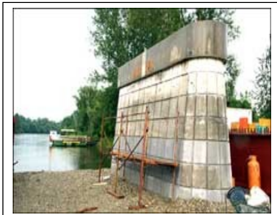
VIEW TO THE BRIDGE COLUMN ON THE SIDE OF ST.MARTIN
