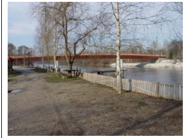
VIEW TO THE BRIDGE FROM CROATIAN EAST SIDE
