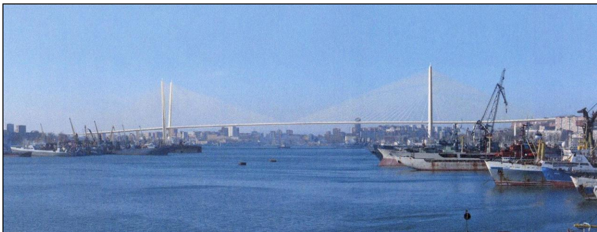
SIDE VIEW TO THE CABLE STAYED BRIDGE OVER GOLDEN HORN IN VLADIVOSTOK, RUSSIA.
