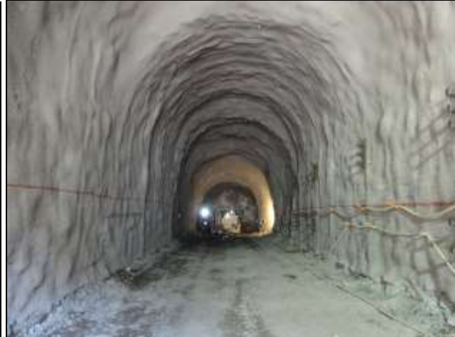
CONVENTIONALLY EXCAVATED TUNNEL VL1
