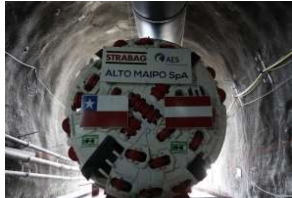
HARD ROCK OPEN TBM FOR L1 TUNNEL
